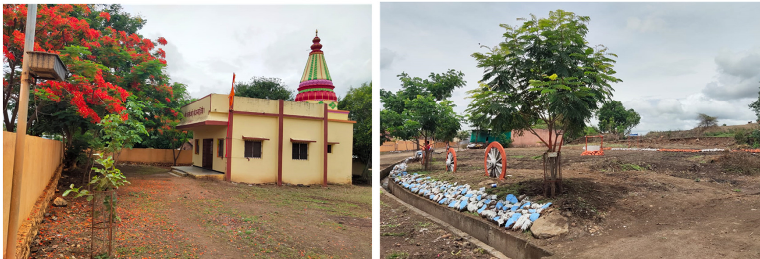
BFL's Infra work changed the view of village
