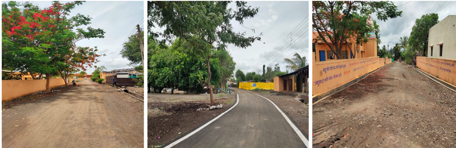
Construction of Internal Gutters and Tree Plantation
